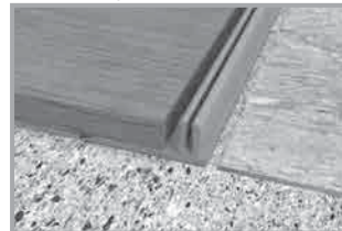
C: Flooring fitted to base
