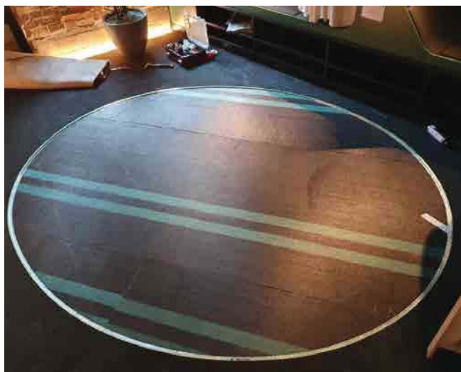
Profile installed against template.
