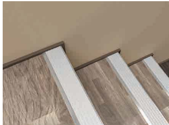
Example: AN15 Polished Aluminium stair nosing with LRV 75.55 installed with a Castellated PVC Infill in White, with LRV of 84.22 on a flooring with an LRV of 32.
