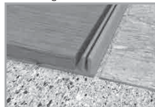
C: Flooring fitted to base
