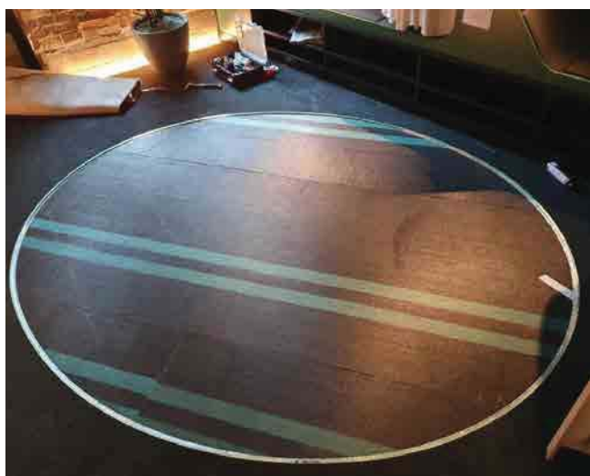
Profile installed against template.
